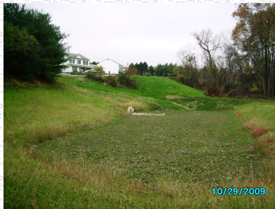
The above picture shows the completed retrofit.
