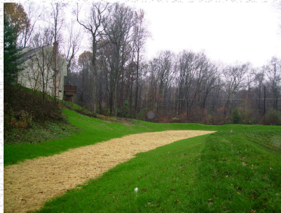
Photo shows the completed facility.
